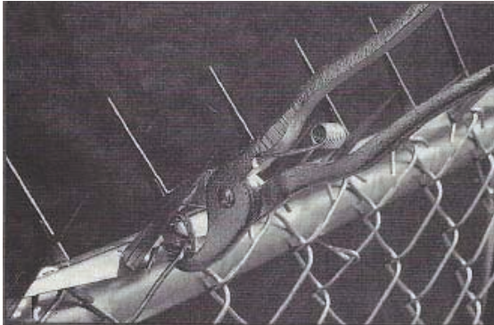
Position loaded Hog Ring Pliers around fence fabric and Ultra-Barrier. Compress pliers until Hog Ring is firmly seated.
